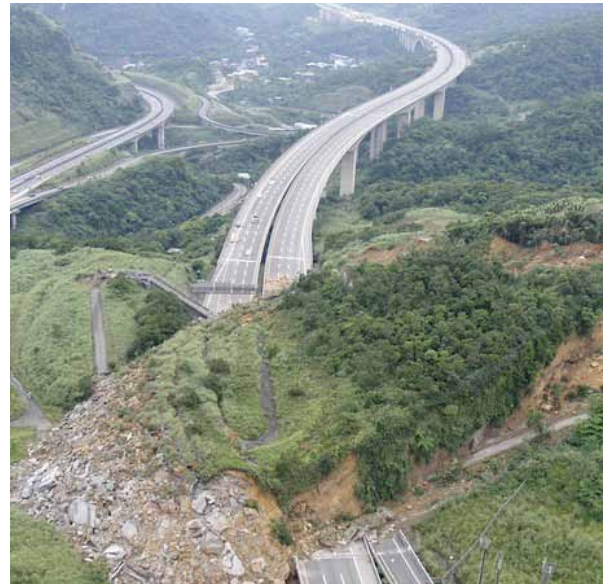
Top: Freeway 3 in Taiwan after a landslide, 2010 (Photo: REUTERS/National Airborne Service Corps) Creative Commons, Flickr Bottom: Hurricane Sandy floods the streets of New York, October 2012 (Photo: Renanit Avitan Fein)
